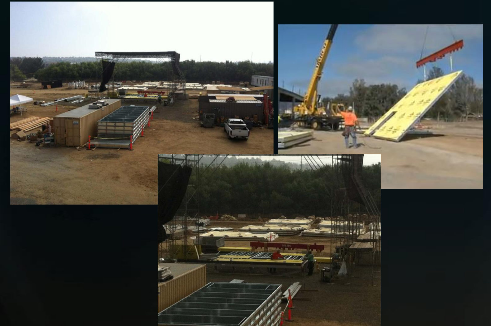
Panel Prefabrication at Hospital in Temecula, CA
